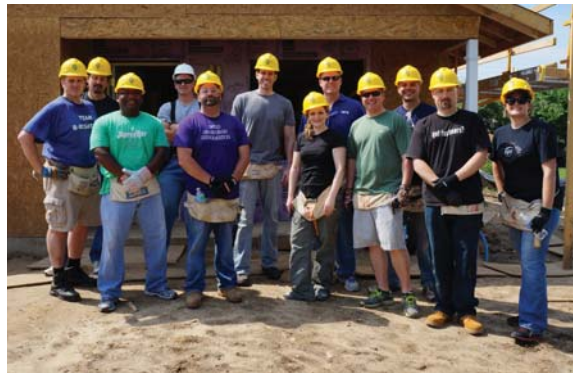
FIELD FASTENING CO. TEAM MEMBER VOLUNTEERS POSE OUTSIDE THE HABITAT FOR HUMANITY HOUSE THEY ARE SPONSORING AND BUILDING IN MACHESNEY PARK AFTER THE FRAMING OF THE EXTERIOR WALLS WAS COMPLETED. THE RESIDENCE SHOULD BE READY FOR MOVE-IN BY AUGUST.
