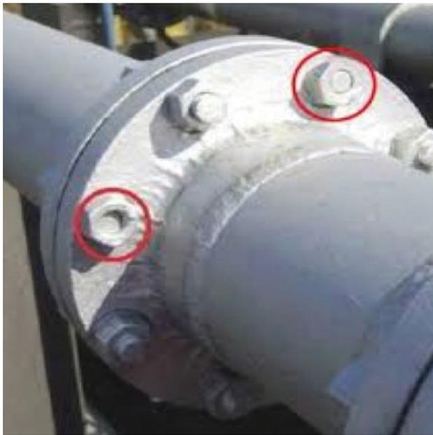
FIGURE 2: EXAMPLE OF A PIPE FLANGE WITH FAILED JOINTS
