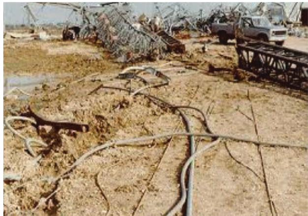
FIGURE 1: CRUMPED STRUCTURE AND GUY WIRES OF THE COLLAPSED TOWER
