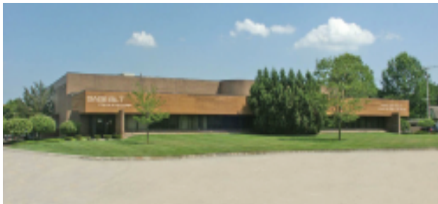
Gage Bilt's Clinton Township facility
