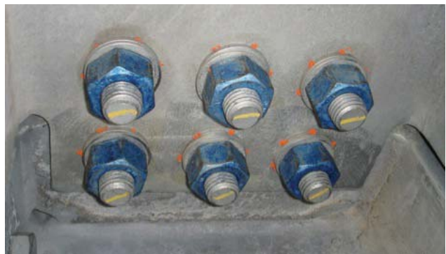
Figure 3: Squirter DTIs Make Installation and Inspection Easy
