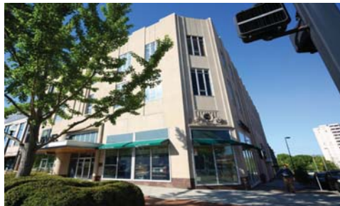
MARTIN SUPPLY HEADQUARTERS, ALABAMA
