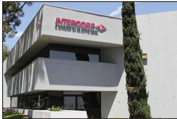
Intercorp's headquarters in Los Angeles, CA
