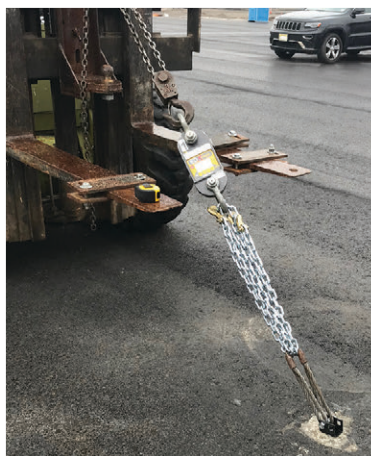
PULL TEST USING FORKLIFT
